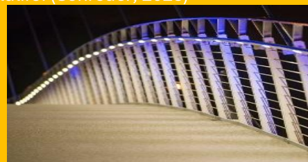
Figure 1: Smart and Adaptive Lighting (Schreder, 2025)
